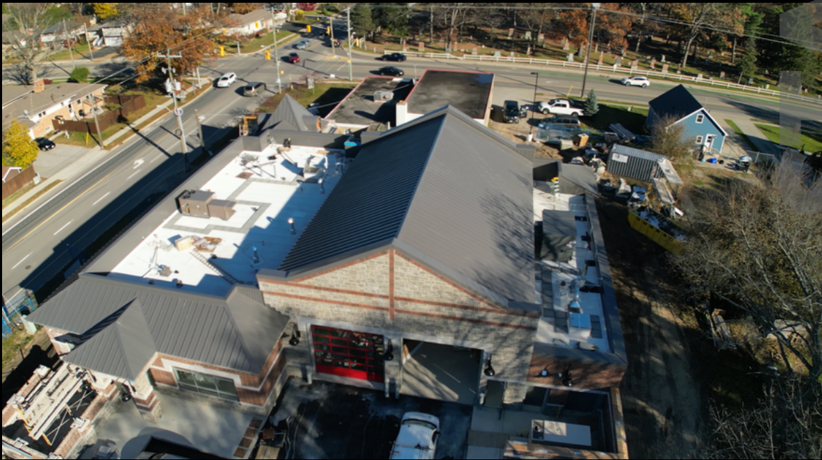
Sarnia Fire Station
