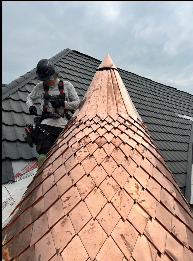
Diamond Copper Tower | Brampton, Ontario
